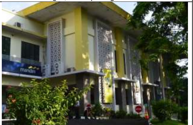
Figure 6. Smart Building implementation in the UNS Inn
