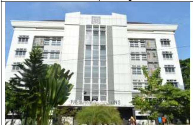
Figure 5. Smart Building implementation in the Post Graduate Building UNS
