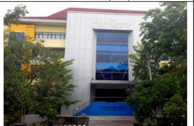
Figure 4. Smart Building implementation in the Building E, Faculty of Agriculture UNS
